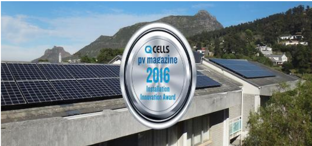
Photo02: 2016 installation innovation award for the maxx Grimley School project
