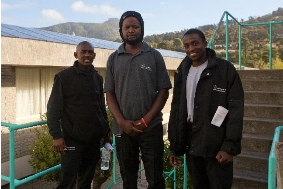
Photo 01: maxx-team installer SolarpowerPB in front of the system at Grimley School, Hout Bay
